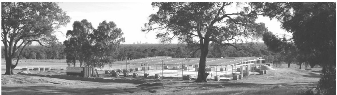
The slab has now been poured for the traditional Tibetan temple.
